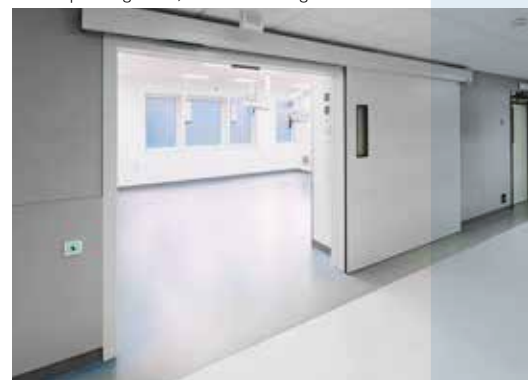
▲ Sweden - Eksjo: Operating Block, Hermetic Sliding Doors
