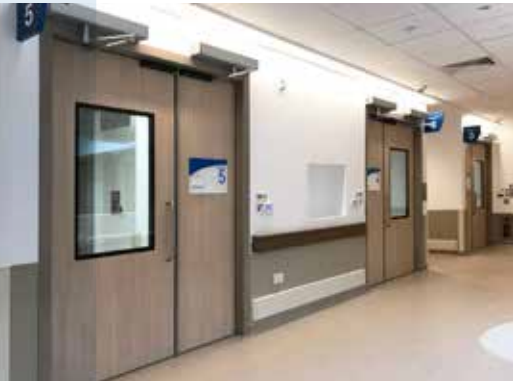
▲ Singapore - Sengkang: Isolation Rooms, Hermetic Swing Doors
