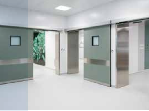
▲ Algeria - Constantine: Operating Block, Hermetic Sliding Doors
